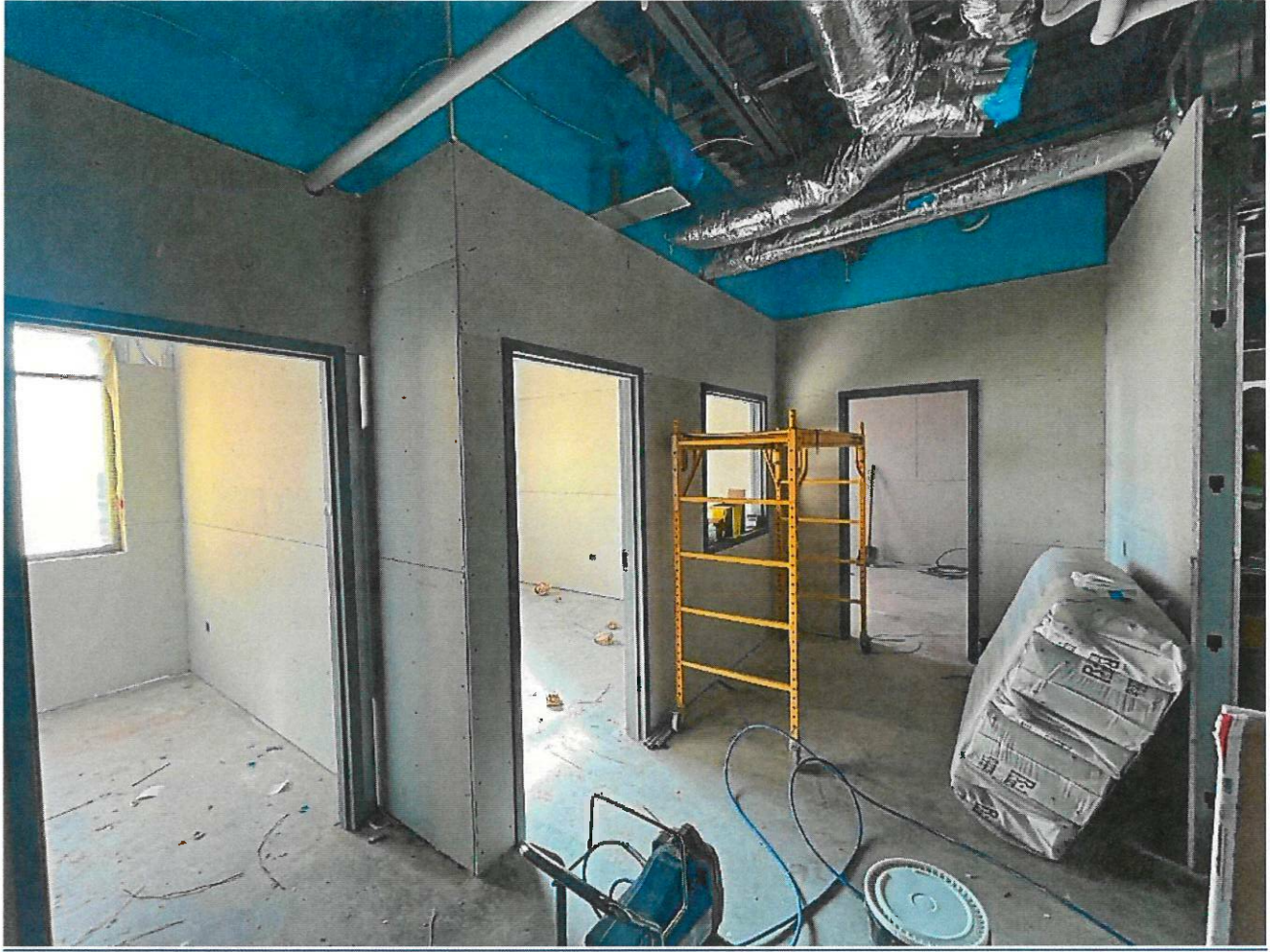
Progress on the interior.
