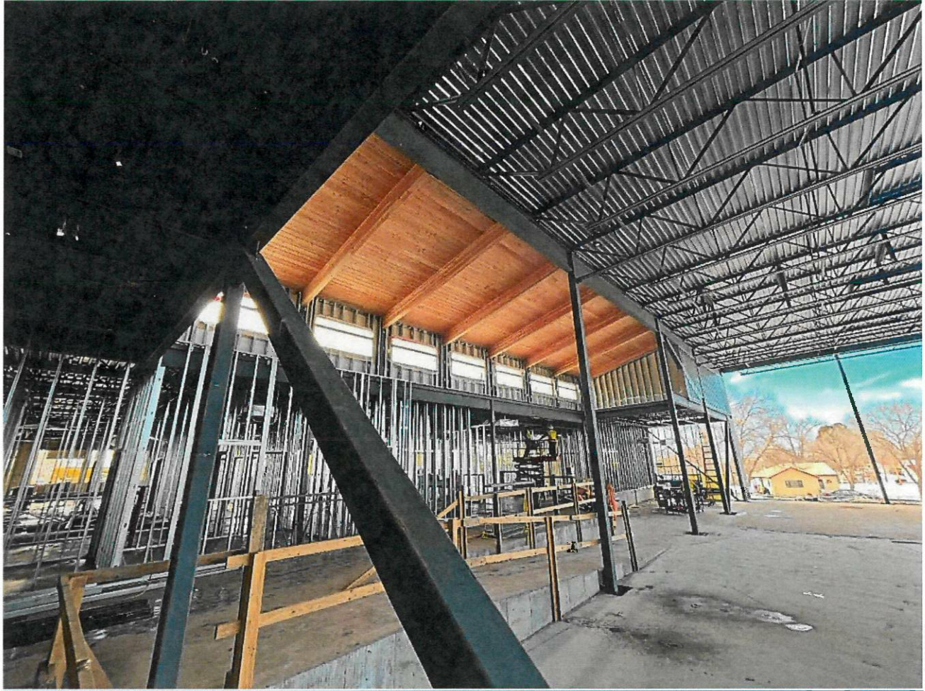
Tongue and groove, glulams, and clerestory openings framed in.
