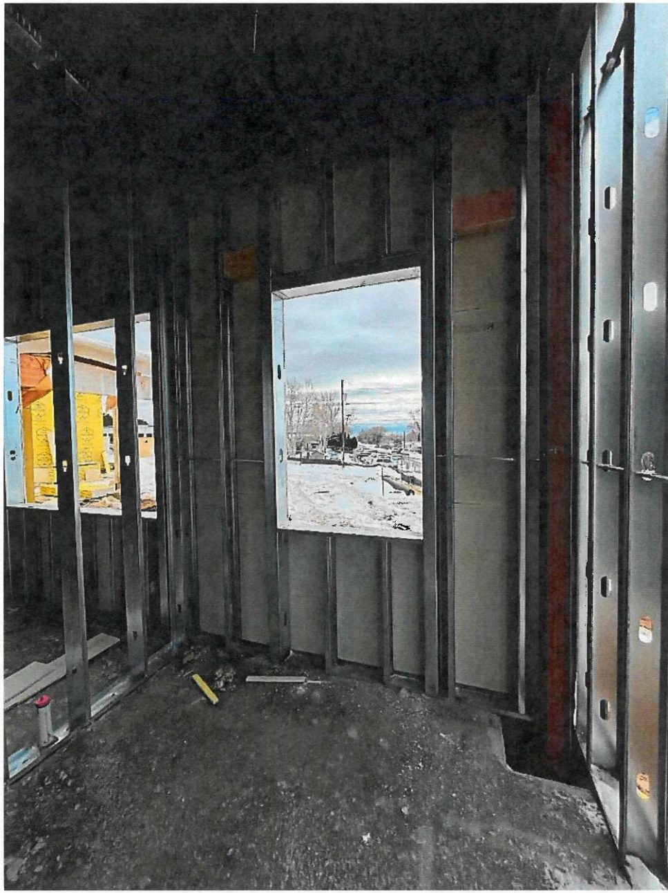
Interior framing and exterior sheathing complete in the Administration wing.
