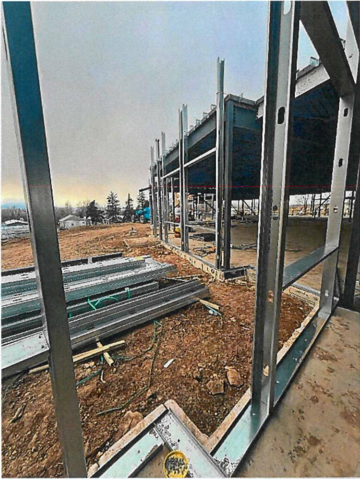
Exterior framing installation on the south side of the building.
