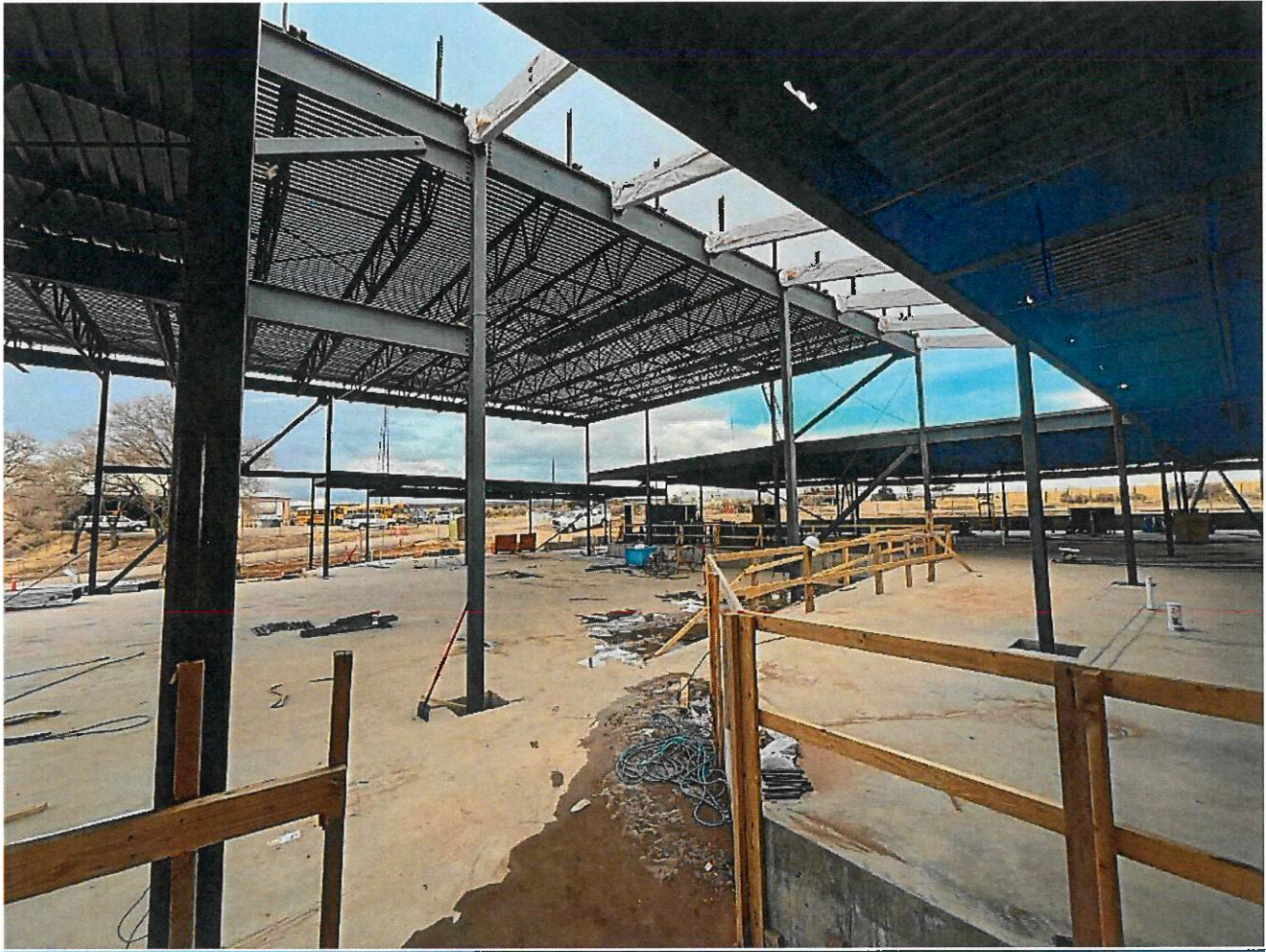
The clerestory section between the main corridor and the gymnasium.
