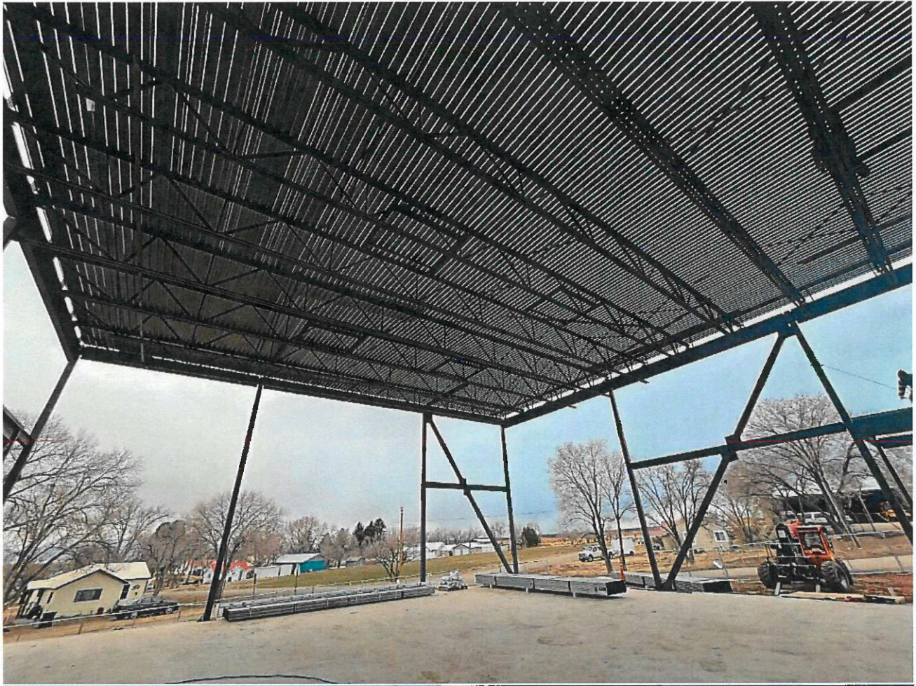
Steel decking in the gymnasium.
