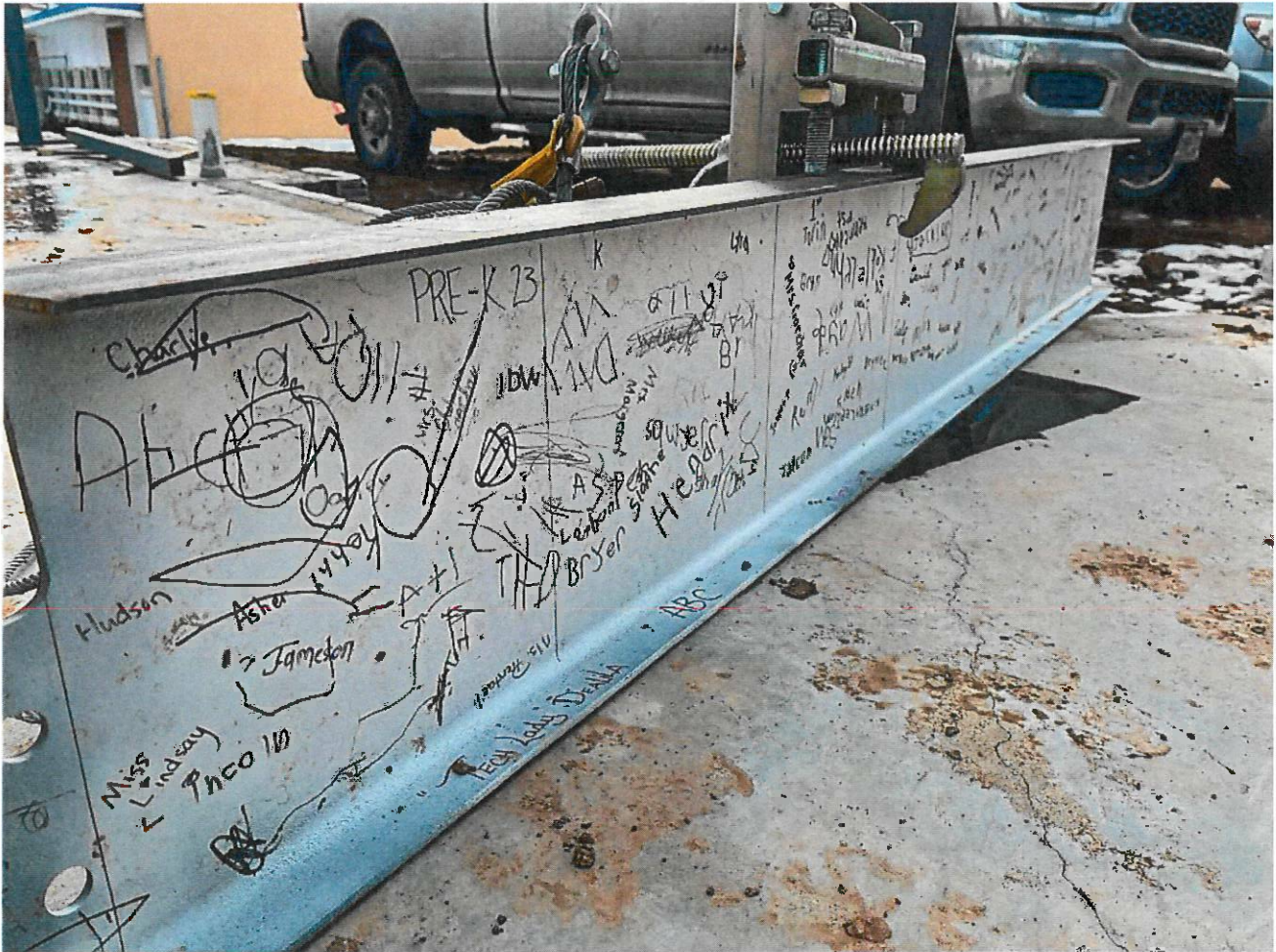
The special beam has been signed by students and staff and will be set into place.
