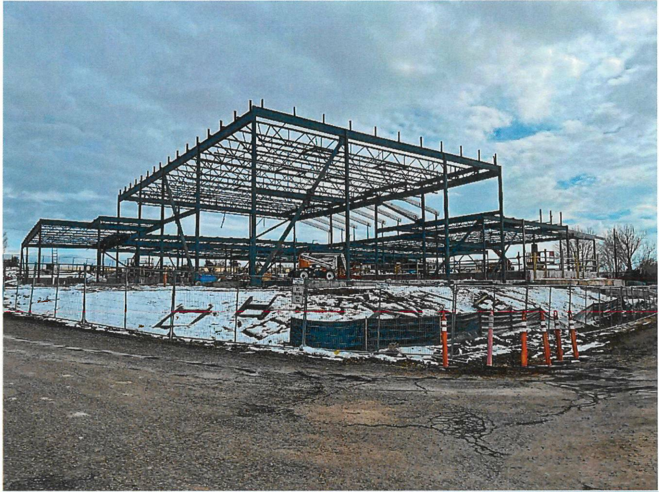
Most of the steel for the building has been set.
