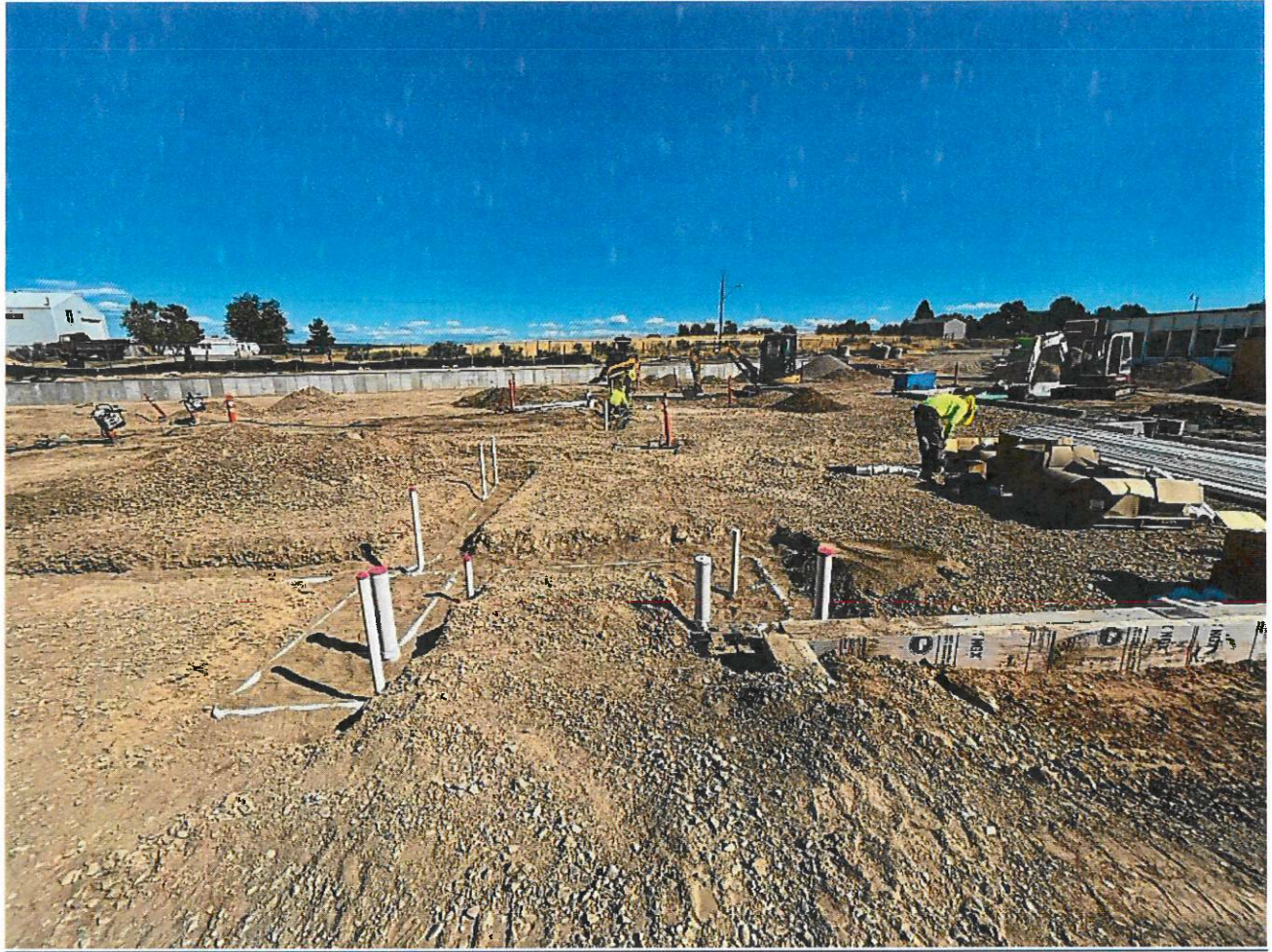
Underground electrical and plumbing installation in the Elementary offices area.
