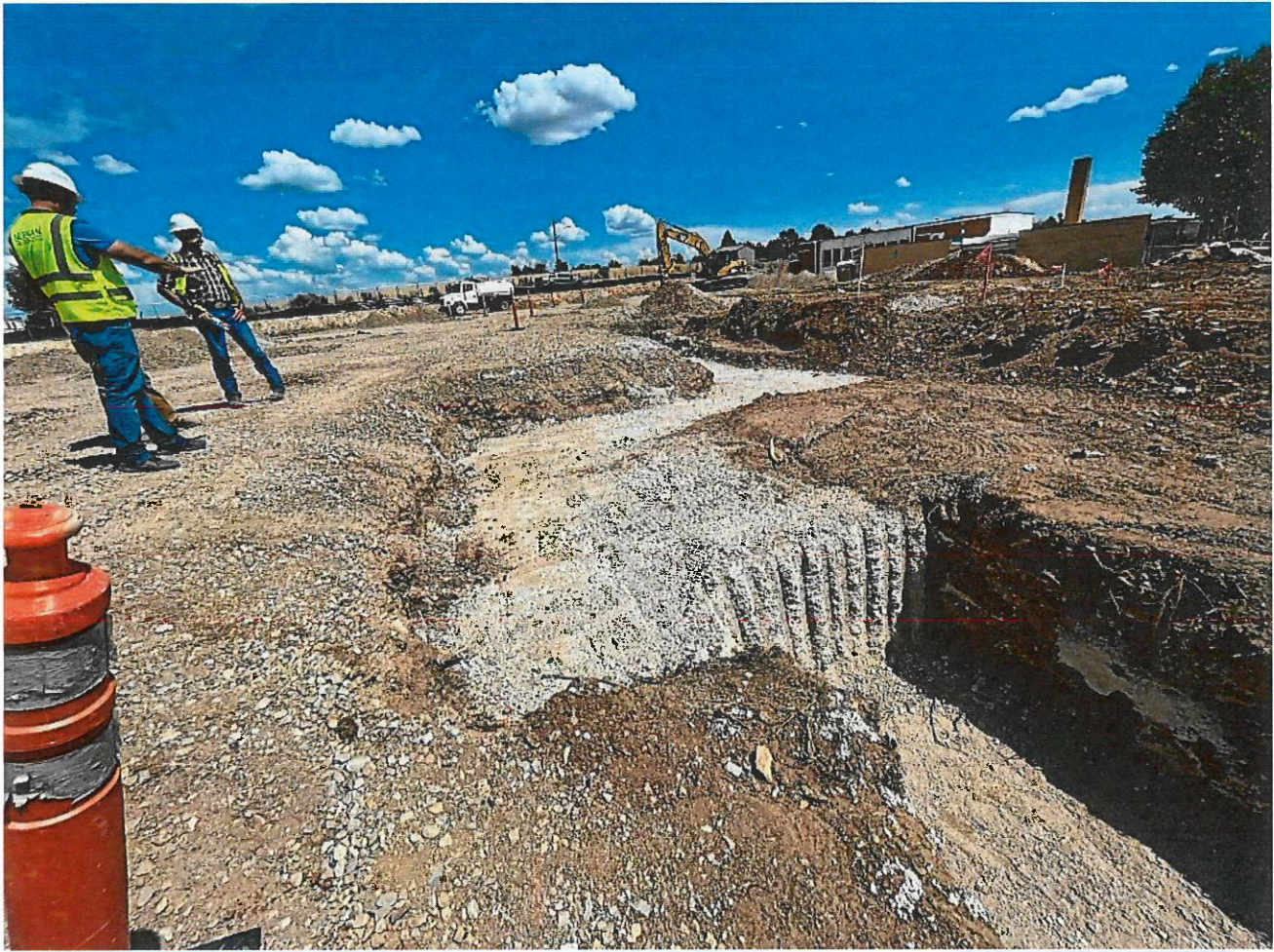
Closeup of the placed flowfill.
