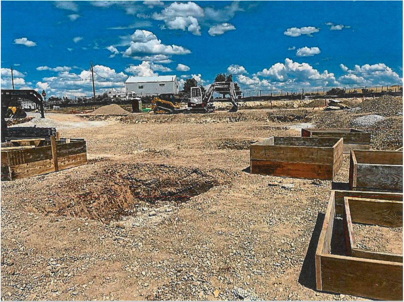
Interior pad footings being excavated and formed.
